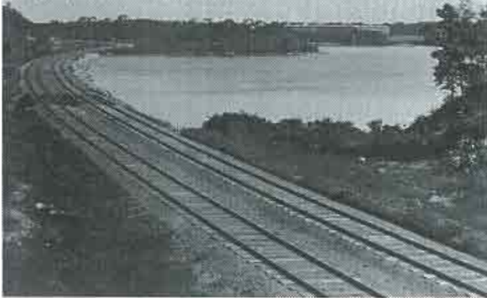
Looking east along the rails in Cedar Lake Park, note that the trail right-of-way presently crosses what used to be the lake. See the old ice house on the far-eastern side.
